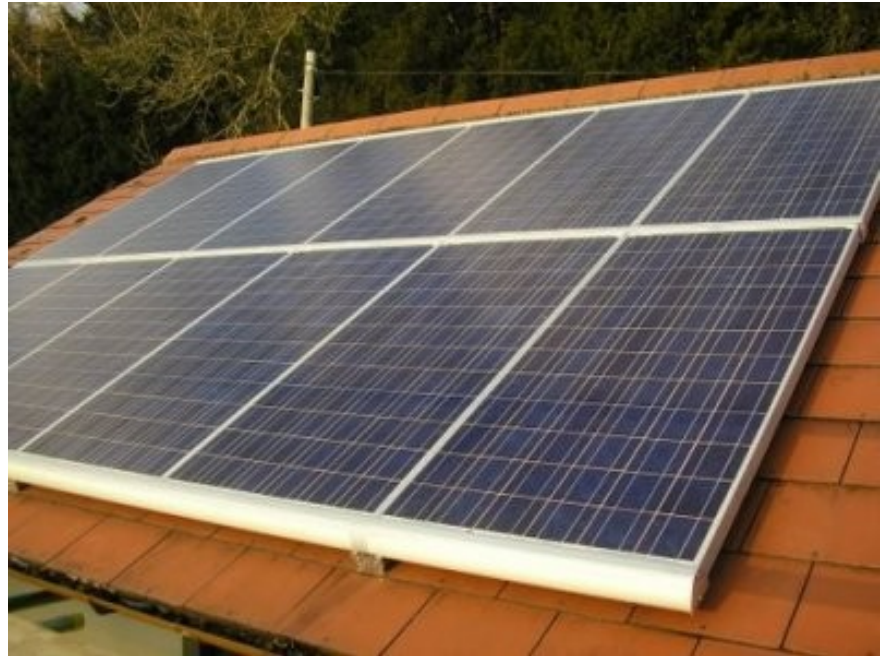
A grid -tied roof mounted system by www.greensystems.co.uk
